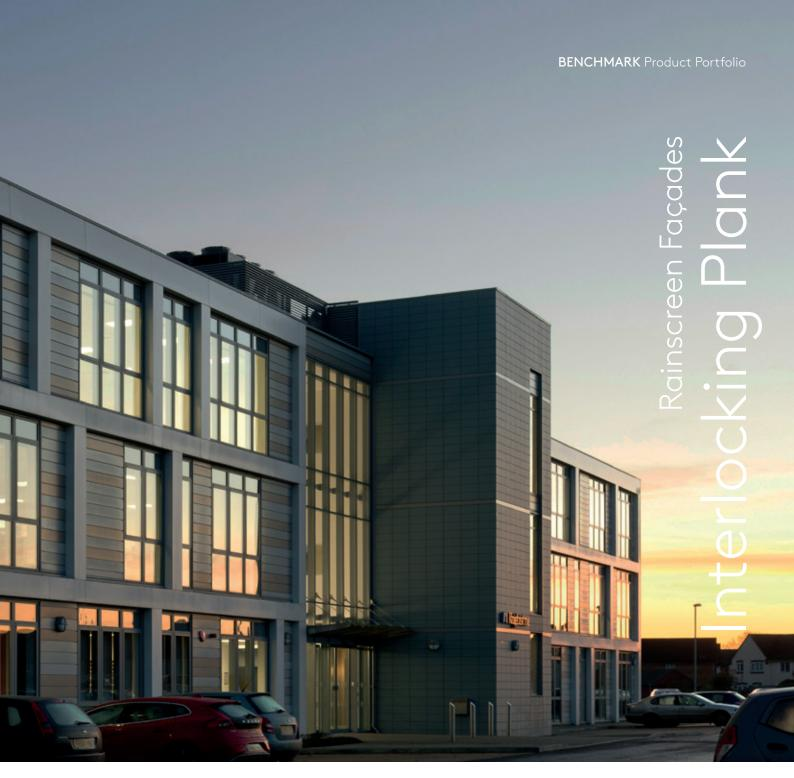
Interlocking Plank is secret-fix with flexibility in joint and face widths creating slim, linear designs. This system produces striking lines on buildings creating a bespoke look.
