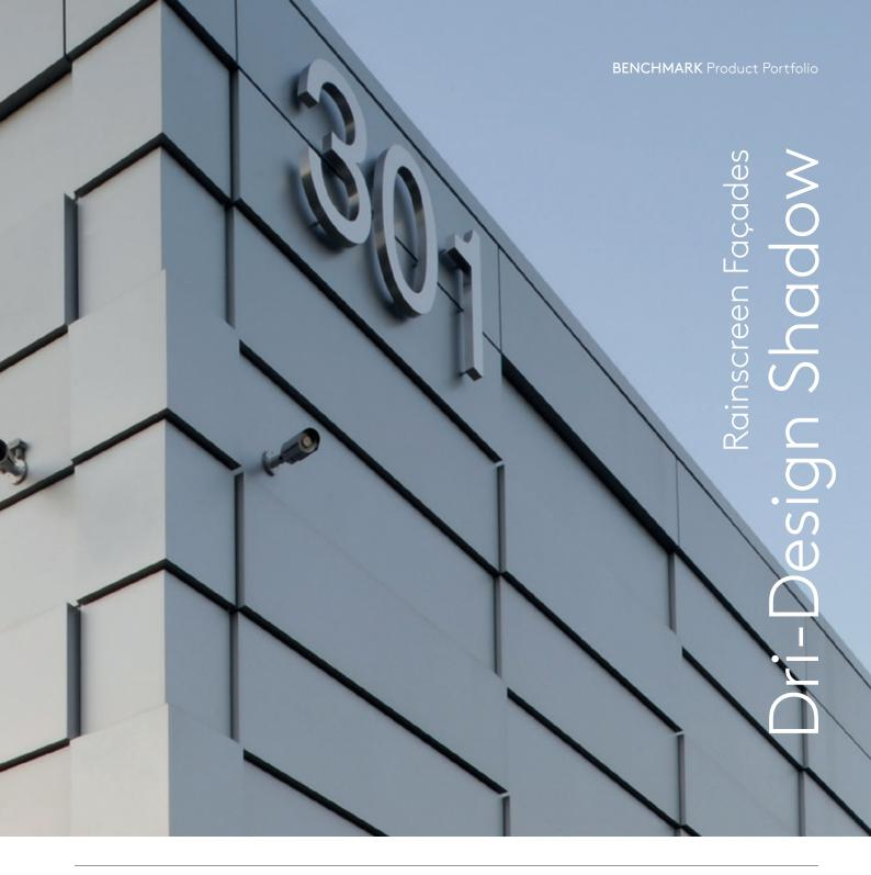
Dri-Design Shadow cassettes let you add depth and definition to any architectural design. Individual panels can be extended at varying depths to create texture or a dynamic variation in patterns, all while keeping the substrate and weather barrier in the same plane.
