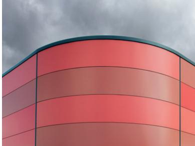
To complement the super smooth aesthetics of the Evolution range the panels are available in a large colour palette in three collections, Kingspan Altaris, highly polished and two tone colour coatings; Kingspan Textured, coarse rendered effect coatings; and Kingspan Spectrum, smooth solid, metallic and diamond coatings.
