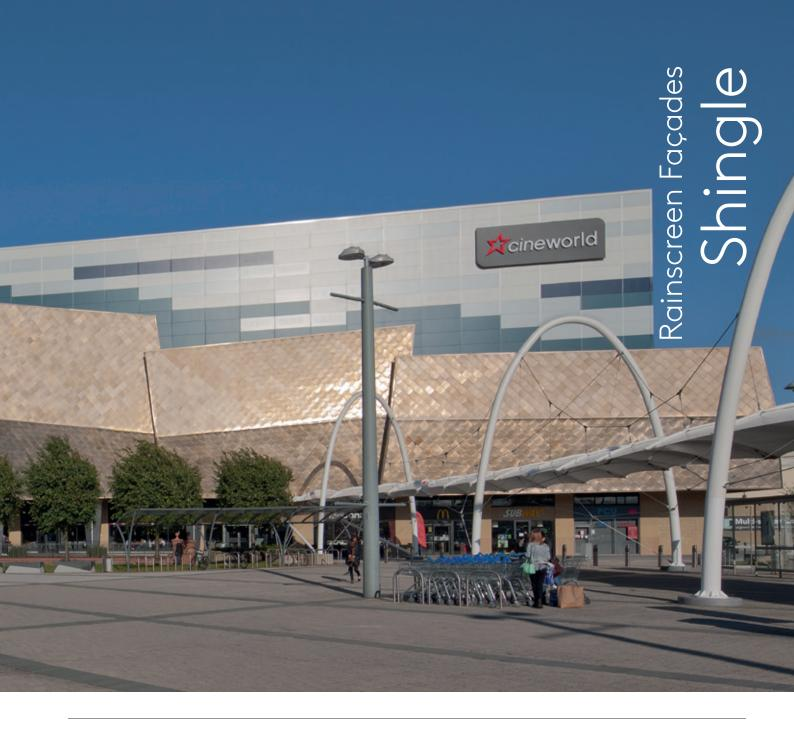
Shingle is available in various sizes and polygon shapes, providing a distinctive façade solution. This is a cost-effective method as a secondary support/railing solution is not required as standard.
