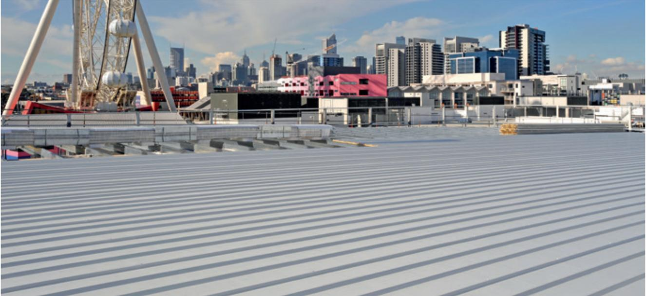
**Kingspan Foilback is designed for applications with suspended ceilings that require thermal regulation compliance (air conditioned space) and used in combination with additional insulation methods or for applications where a prefinished steel internal liner is not required.**
