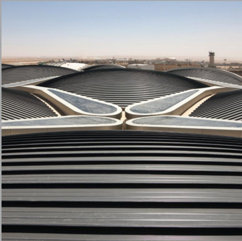
A unique high performance standing seam roofing system offering premium aesthetic and that is zipped on-site to create a weathertight solution.
