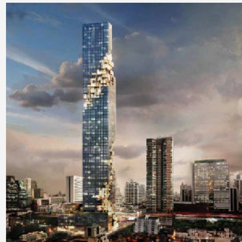
Commercial Building/ Hotel
